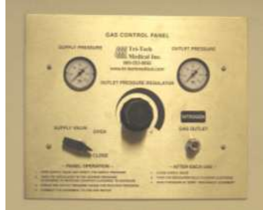
NP100 – Nitrogen Gas Control Panel Shown
