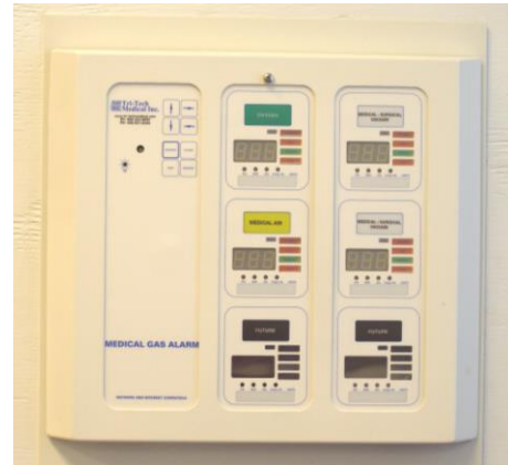
Area alarm shown is 4 gases, and 2 future expansion modules part # DU7OAFVVF
