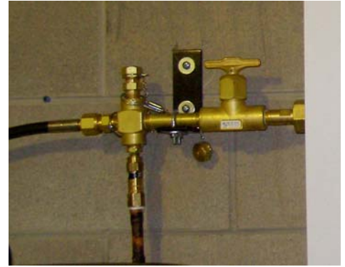
20" header length (Header pictured above accommodates 2 - 72" flexible pigtails for 2 portable bulk vessels + relief valve with pipe away)
