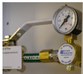
Single port E Z Backfeed™ fitting with Gauge & DISS gas specific demand valve on the right side port shown above Shown above EVU4R2AB2NB3OB4VS 4 valve box with gauges 1/2" Medical Air, 1/2" N 2 O, 3/4" Oxygen, 1" Medical Vacuum
