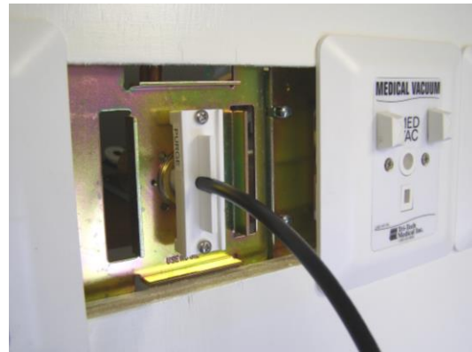
Kit attached to rough-in of medical gas outlet
